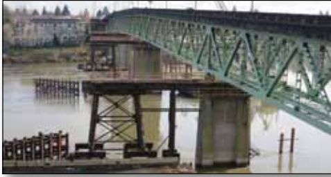
Truss span and detour piers prior to move, 2012
