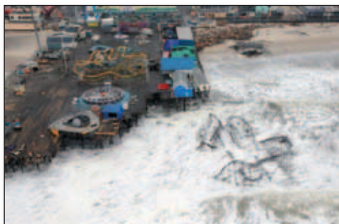
Aerial view of the damage caused by Hurricane Sandy to the New Jersey coast
